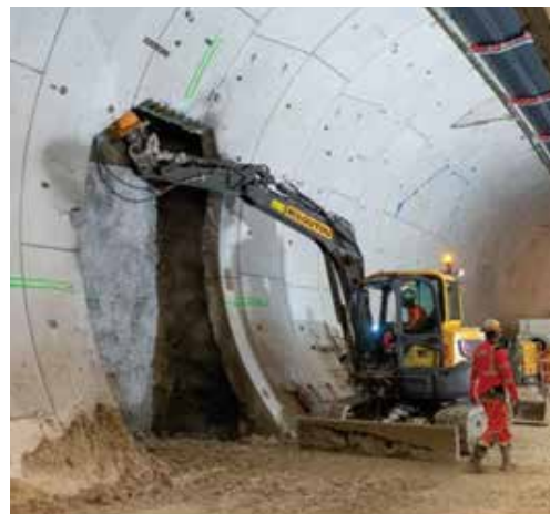
Excavation of cross-passages during tunnel excavation, without any steel structure
