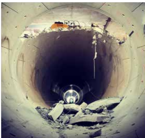
Demolition of the rings in a station without any steel structure.
